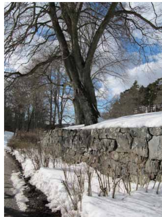
Kallmurad terrassmur i Tollares park.
